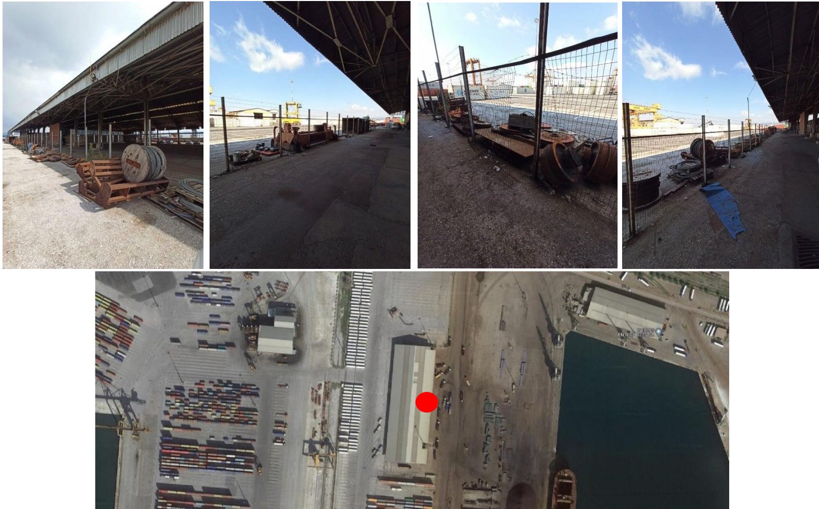
FIGURE 3: POSITION OF ITEMS UNDER THE OPEN SHED IN THE REEFER AREA
